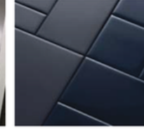
Rear wall textured contrasting blue tile. Large format version behind urinals
