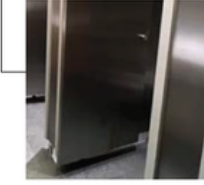
Existing brushed steel doors and cubicles
